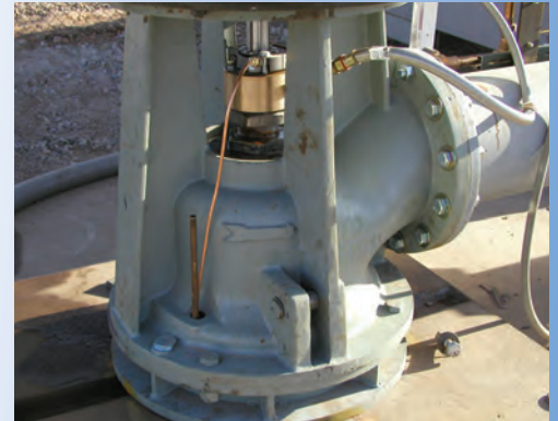
Water Lubricated SXL Bearings Installed In SRP Deep Well Pump, Arizona, U.S.A.
