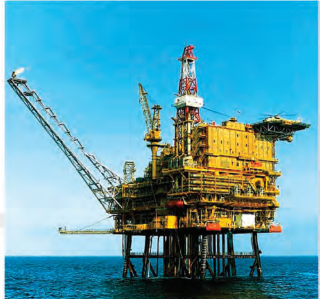
PetroSA's Offshore FA Platform in Mossel Bay, S. Africa
