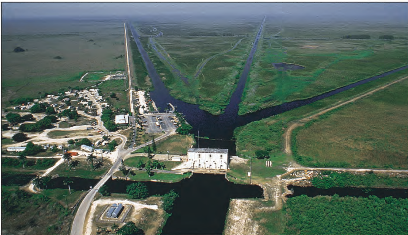
Photo 1. S-9, a retrofitted pumpstation and its environs
