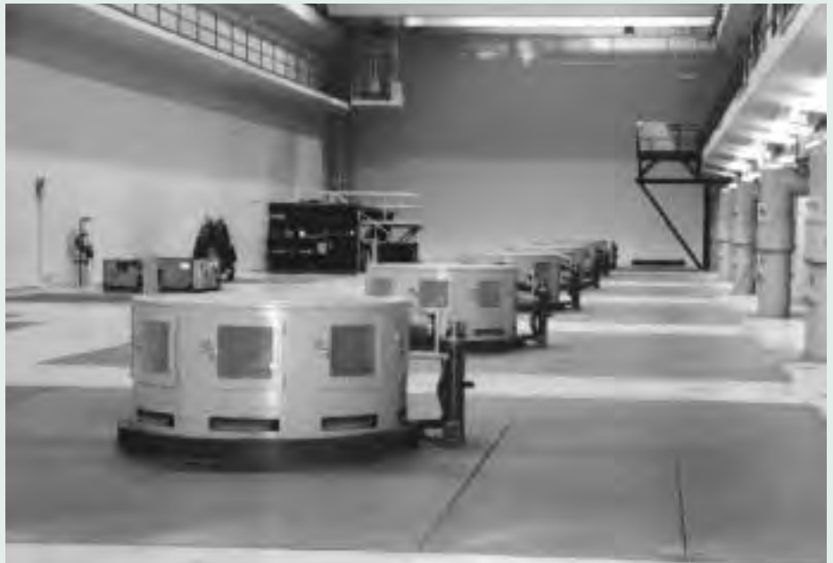
Six 60,000 HP Hitachi pumps at the Havasu Pumping Plant, Arizona.
